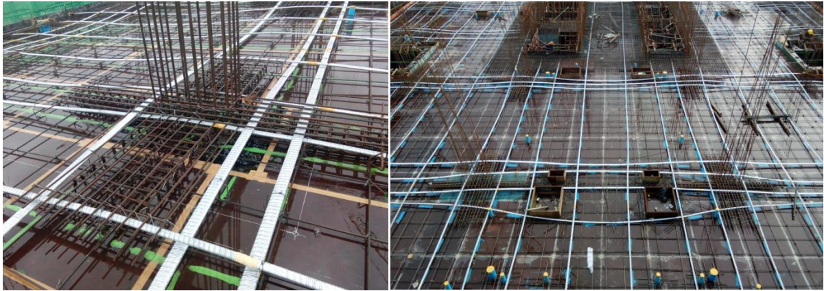
Bonded Post-tensioning system (Flat Slab Design)
